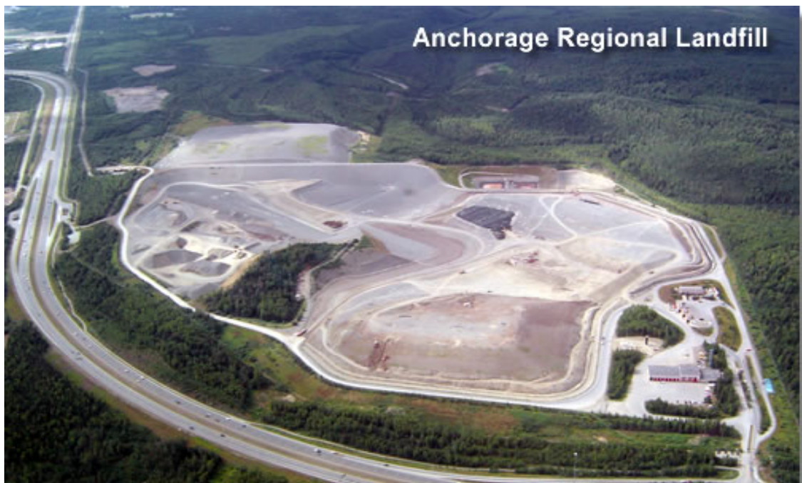
Figure 1: Anchorage Regional Landfill Aerial View
